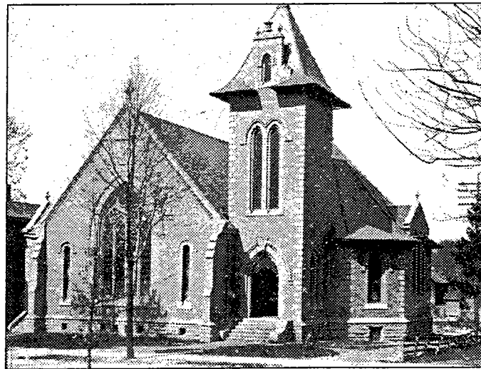
In 1897 the sanctuary was extensively remodelled, the Sunday School room was added, two vestibules and a tower built, stained glass windows installed, and the outer walls were faced with brick.
